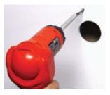
Trill holes into the drywall and insert the drywall mounts into the holes.
